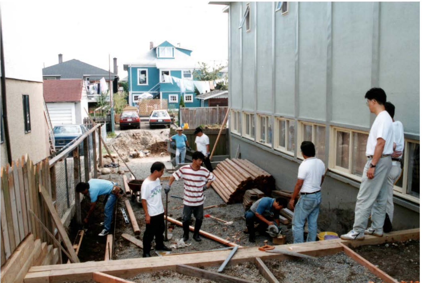
Church Playground Renovation
